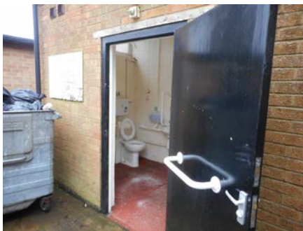
Outside disabled toilet at rear of building
