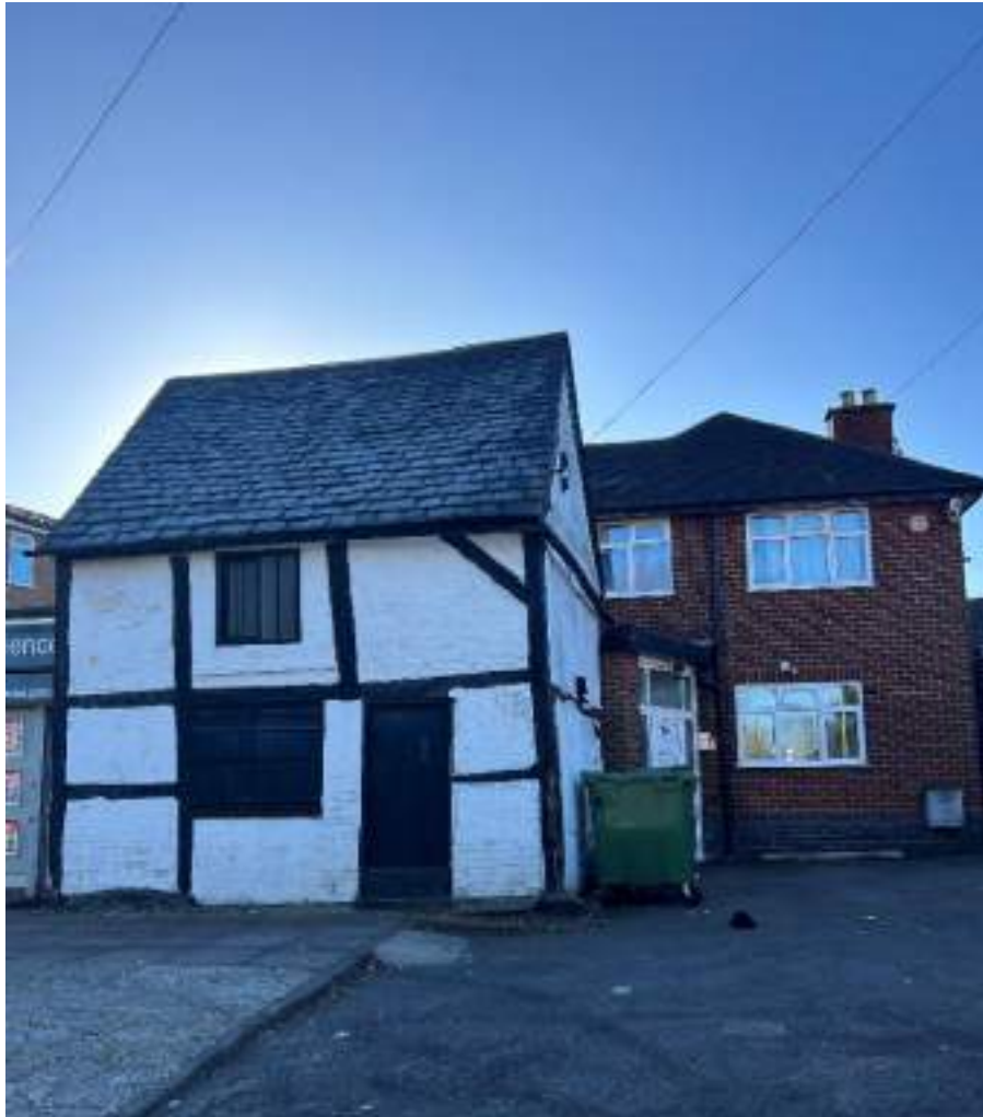
Image 12: Grade II Listed Former Shop with Storage Loft at 266 Braunstone Lane.
