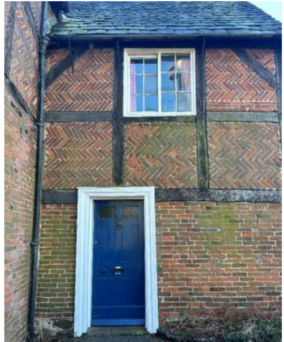
Image 16: The Manor, detail showing herringbone brick pattern, later inserted door and surround and vertical sliding sash window.
